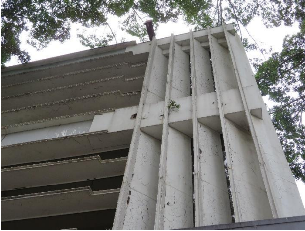
Figure 31 – Detail of horizontal and vertical louvers at the intersection of Cooper Street & Brooklyn Lane.
