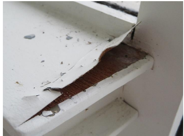
Figure 68 – Detail of horizontal louvre, showing lifted aluminium cladding.
