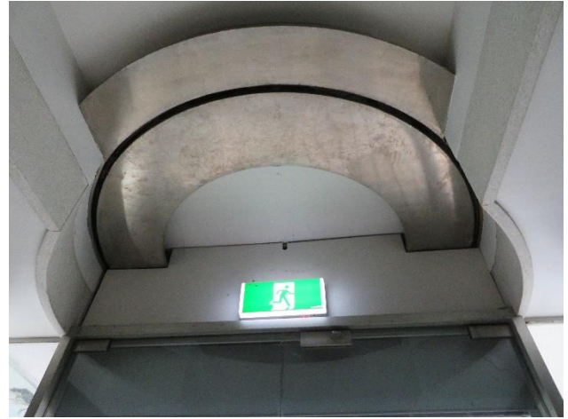
Figure 50 – Ceiling detail above Cooper Street entrance, showing further evidence of removed revolving door.
