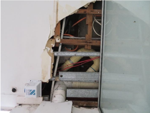
Figure 43 – Detail of services in ceiling and slab structure.
