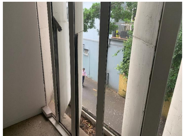
Figure 66 – Detail of louvres from within level 2, showing lifted cladding and paint failure.
