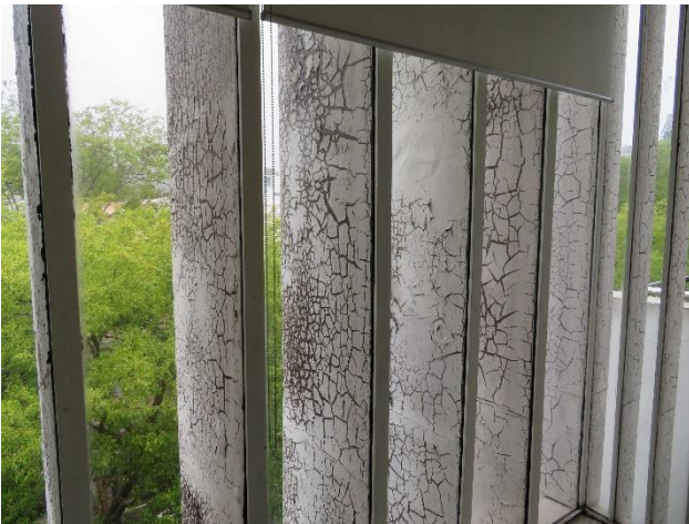
Figure 67 – Detail of vertical louvres, showing paint failure.
