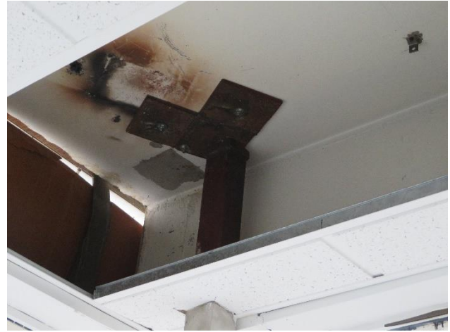
Figure 56 – Detail of later steel structural member.
