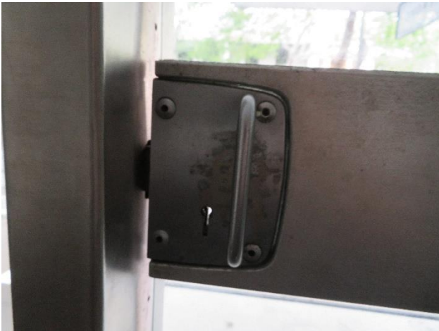
Figure 41 – Detail of original door handle and latch.
