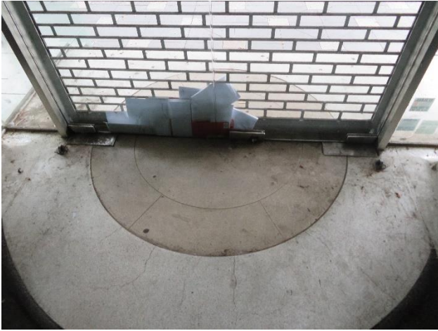
Figure 49 – Detail of terrazzo entrance with evidence of original revolving door.
